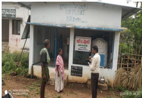
Image 1: RO Plant at Palem Micro Watershed
