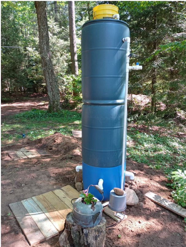
Fig. 5. Field Bio-tower Septic (FBTS) System Installation [28]
