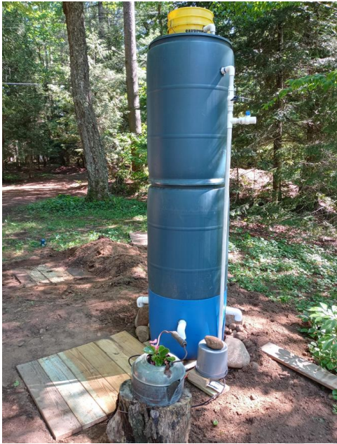
Fig. 5. Field Bio-tower Septic (FBTS) System Installation [27]
