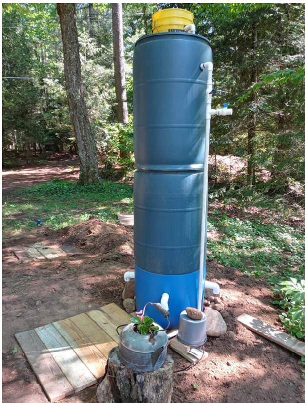
Fig. 5. Field Bio-tower Septic (FBTS) System Installation [27]
