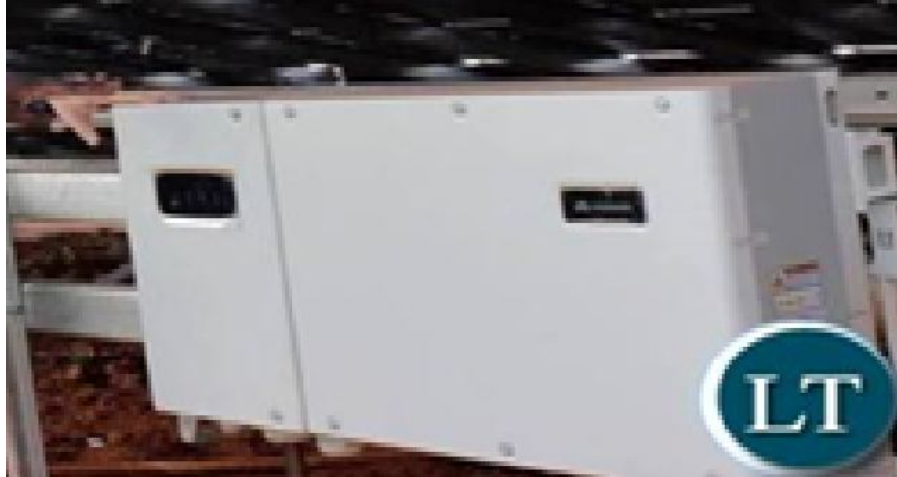
Figure 4.10. Huawei - 480-volt Inverter from Bangweulu Solar Power Station
