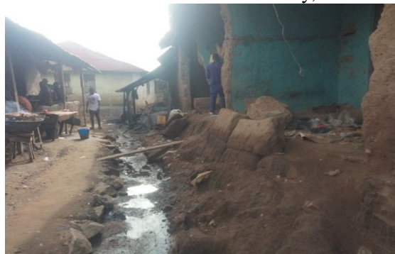
Figure 7: Dilapidated Building Constructed with Mud at Odojoka
