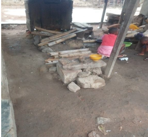
Figure 8: Kitchen Located Outside the Building
