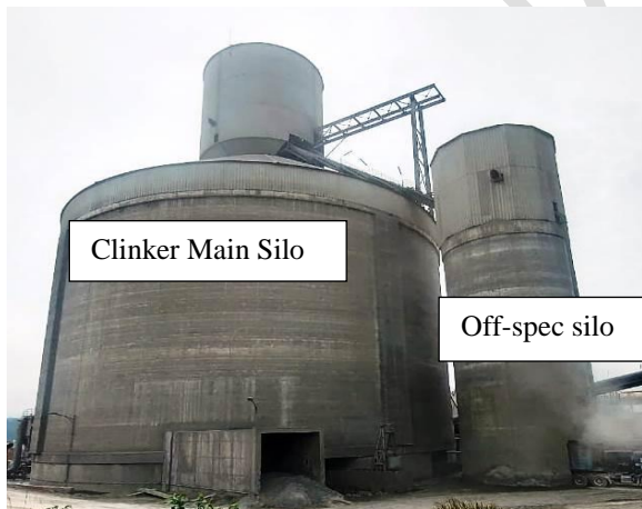
Figure 3: An image of a Main clinker silo and Off – Spec silo in an existing cement plant
