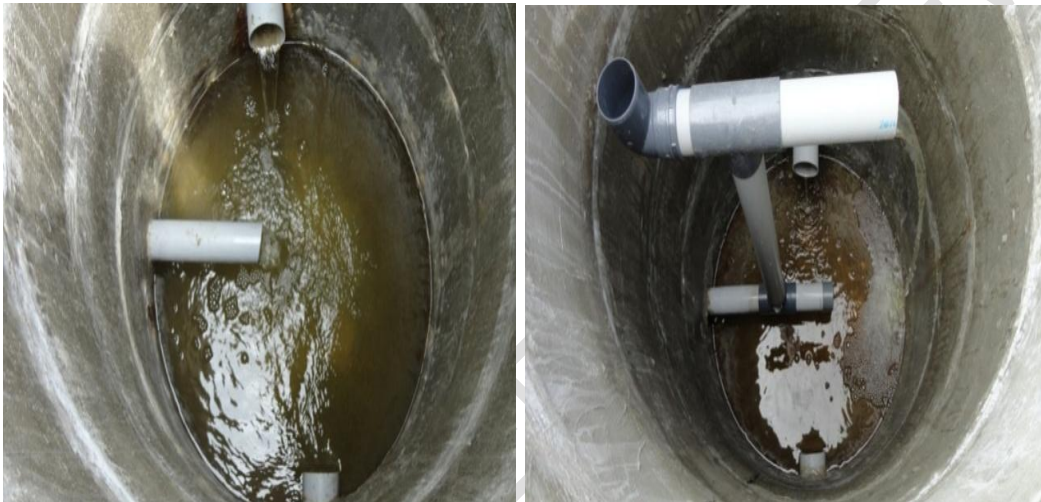
Fig. 2. A view of Conventional and Controlled SSD systems imposed at 50 m lateral spacing at Agricultural Research Station, Gangavathi.
