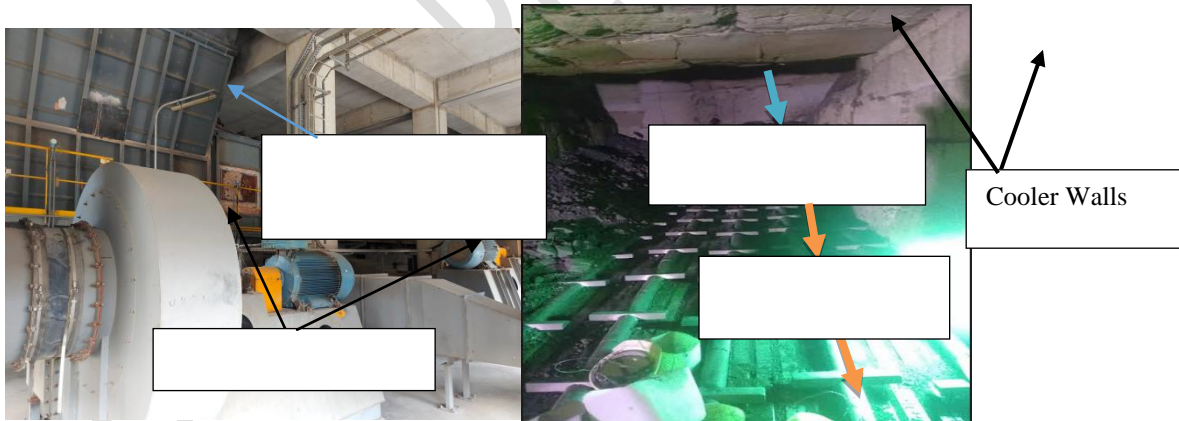
Figure 2a. Suction fan arrangement clinker cooler Figure 2b. Internal arrangement of clinker cooler
