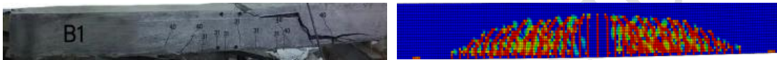
a) Cracking Patterns for Beam (B1) [EXP]. b) Cracking Patterns for Beam (B1) [FEM].
