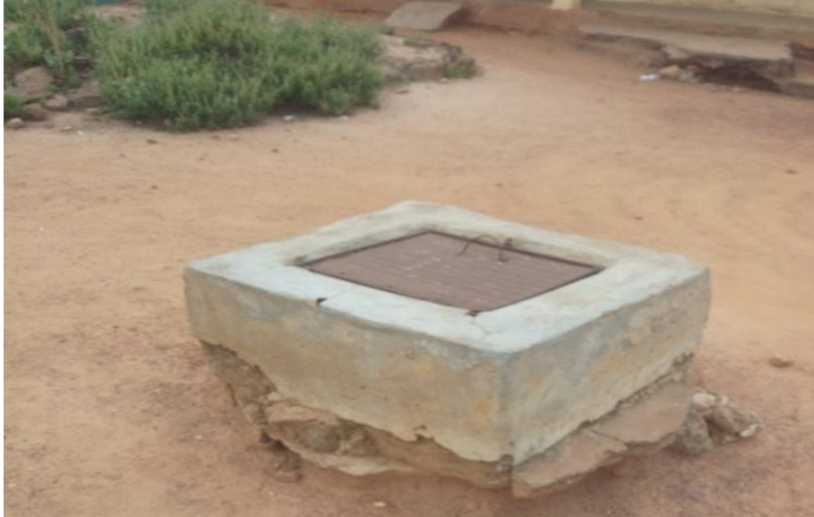
Figure 6: Non-functional covered well in Iju Source: Field survey, 2021
