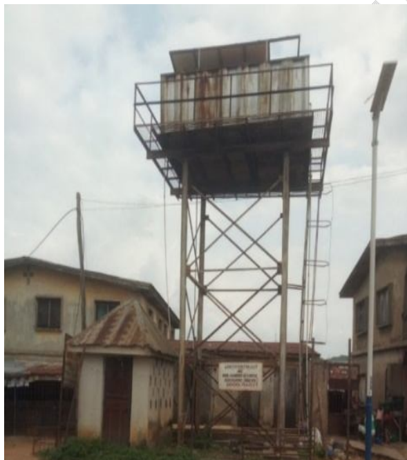
Figure 4: Borehole infrastructure in Iju Source: Field survey, 2021
