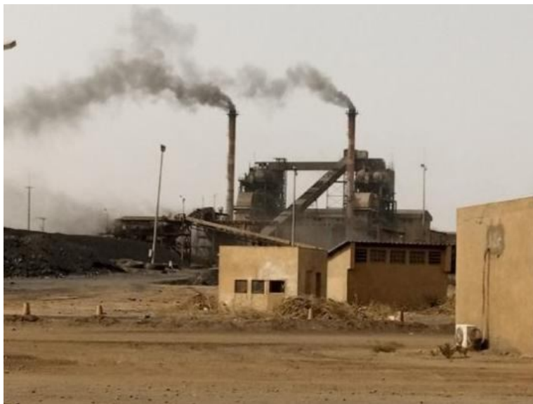
Picture 5: Release of coal dust during mechanical processing activities .
