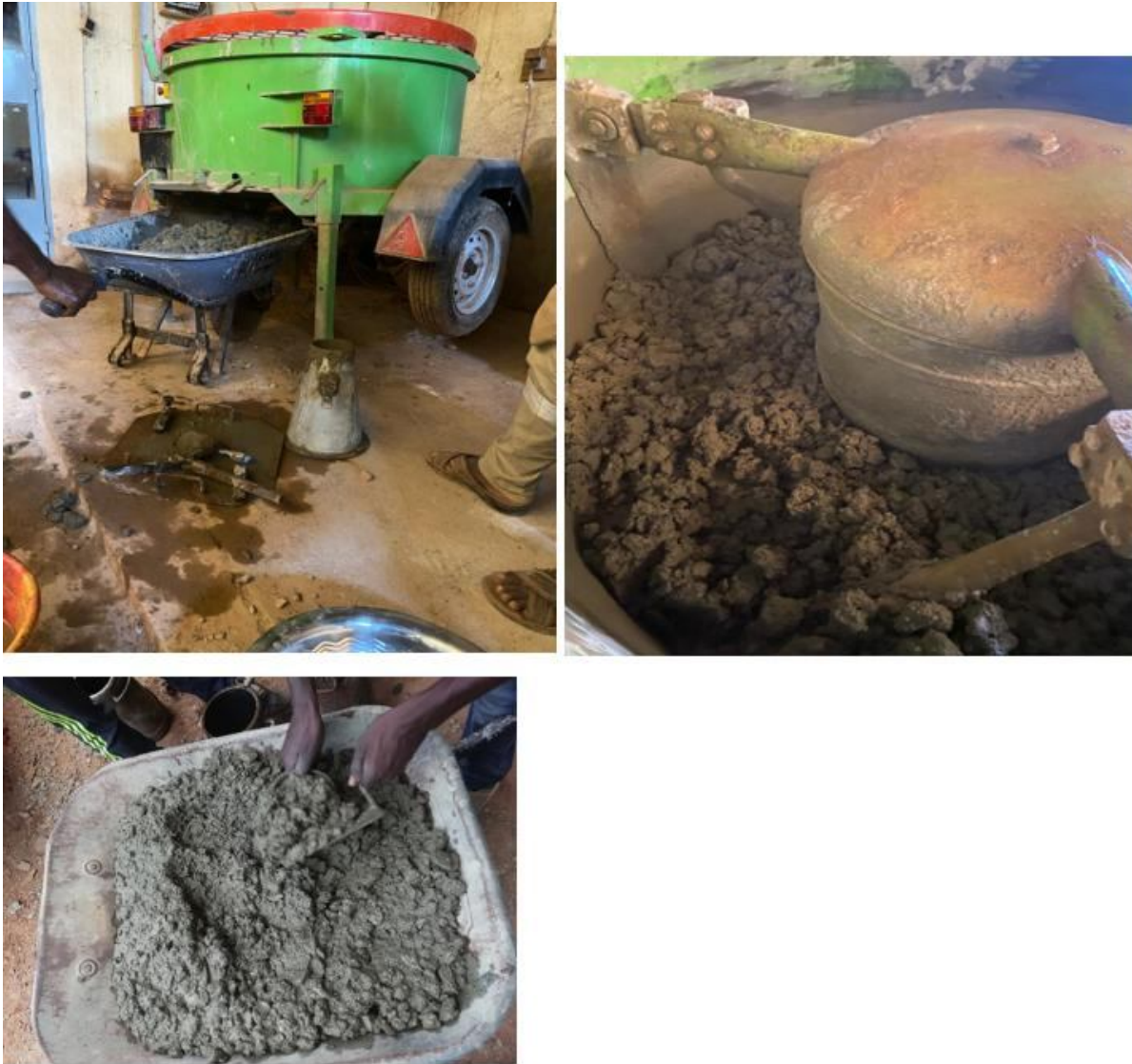
Fig.7.Images of the formed concrete
