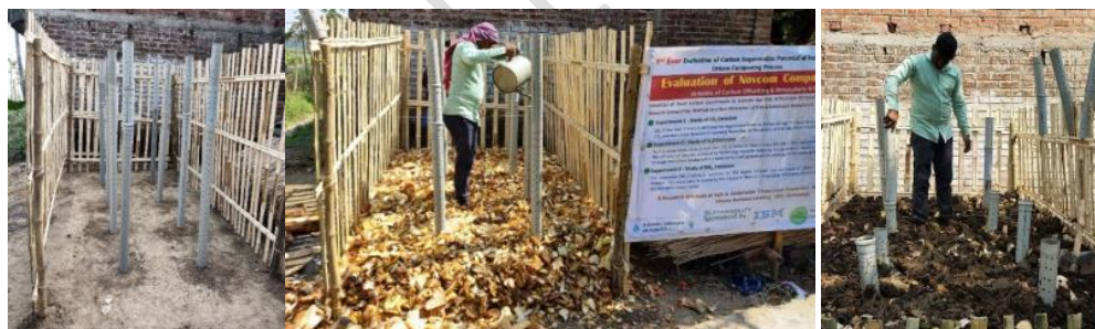
Pic. 1 : Structure for Novcom composting with special perforated pipe for GHG estimation under IBM-IORF Sustainability Project.
