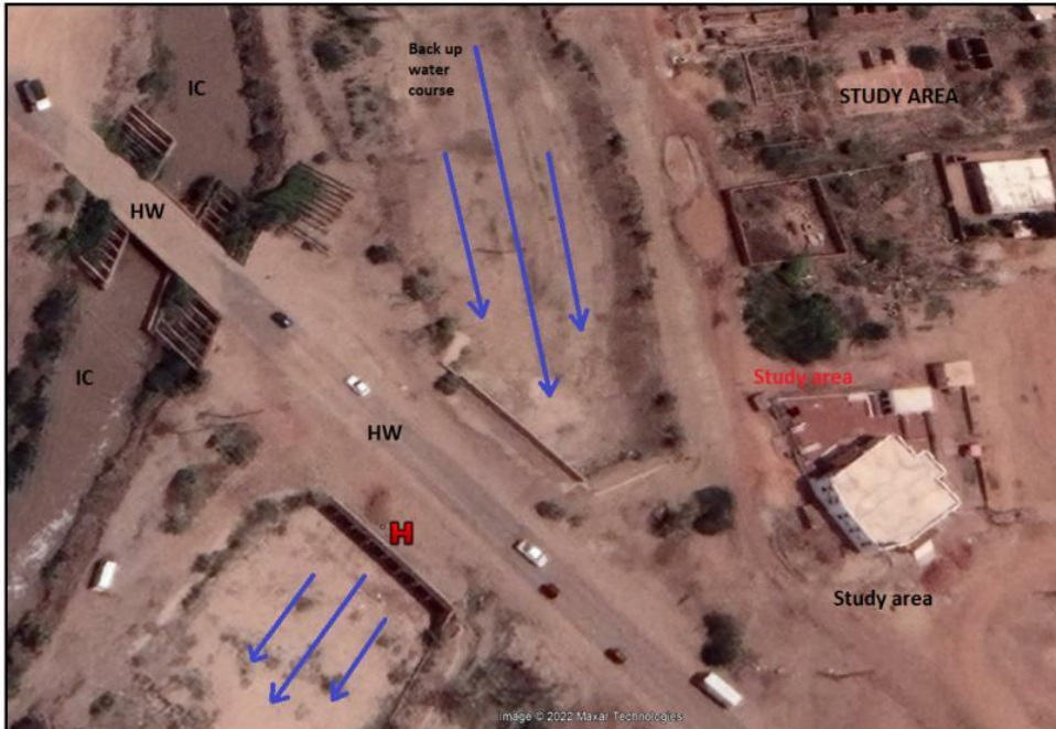
Figure 5, Back up water direction (blue arrows), large culvert (H), irrigation canal (IC) and highway (H).
