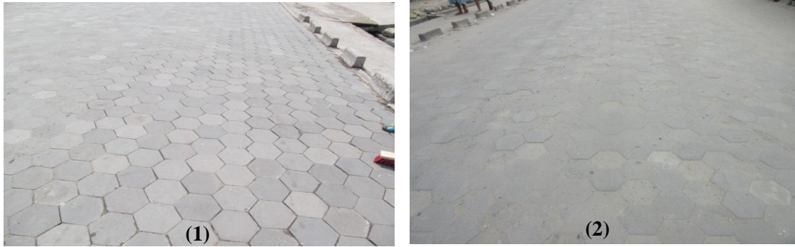
Figure 4. View of the paving stones at the start of installation (1) and after 8 years (2)
