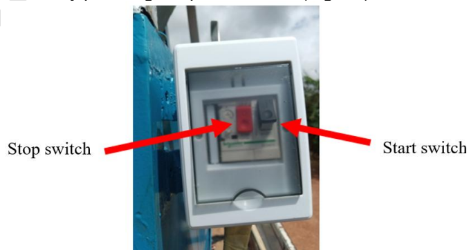
Fig. 11. Device for starting and stopping the roller
