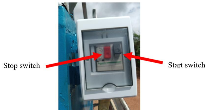
Fig. 11. Device for starting and stopping the roller
