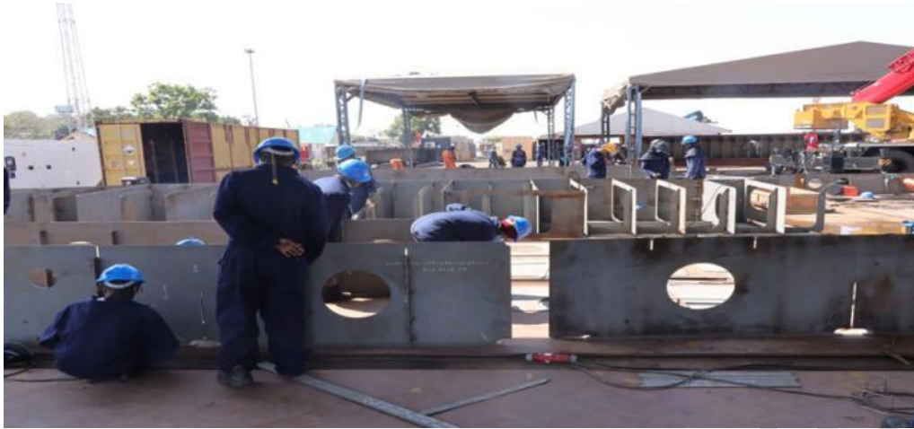
Fig-13 Fabrication of the sections
