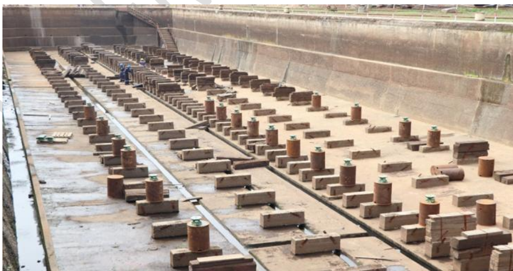
Fig-11 Fabrication of first hull section for MV Uhuru II wagon
