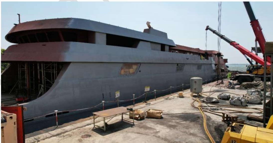
Fig – 17 Construction of bridge deck
