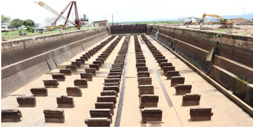
Fig-10 Preparation of dry Dock prior for MV Uhuru II Construction
