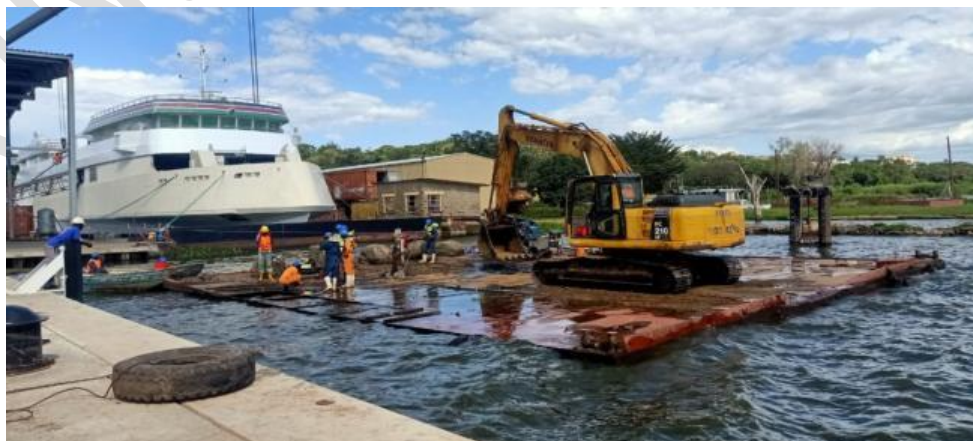
Fig-3 Dredging work at dry dock frontage
