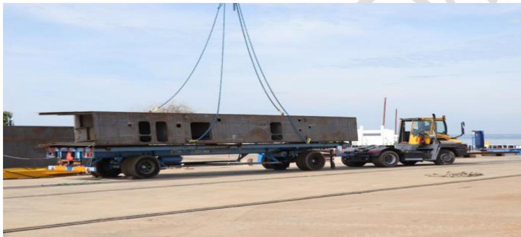
Fig -14 Transportation of sections from fabrication yards
