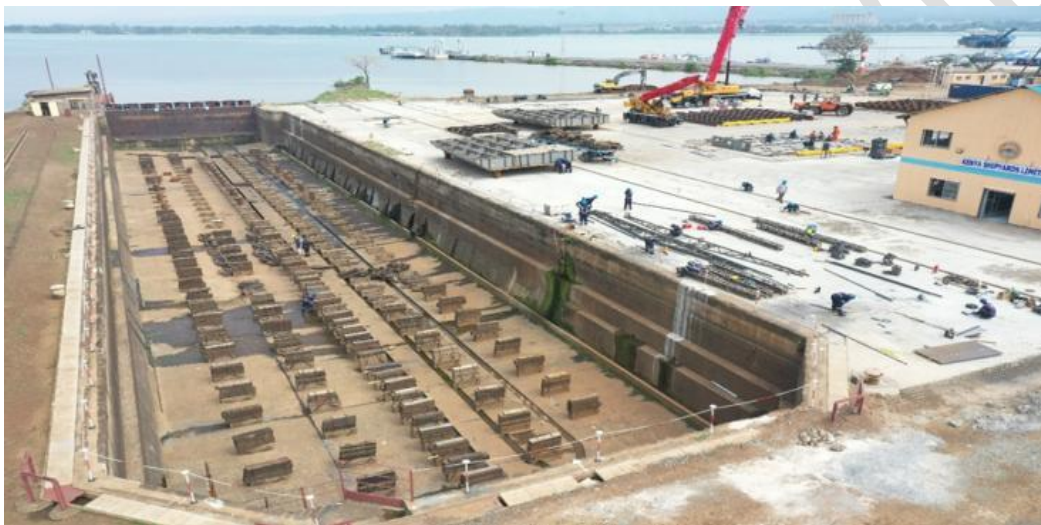
Fig-10 Preparation of dry Dock prior for MV Uhuru II Construction
