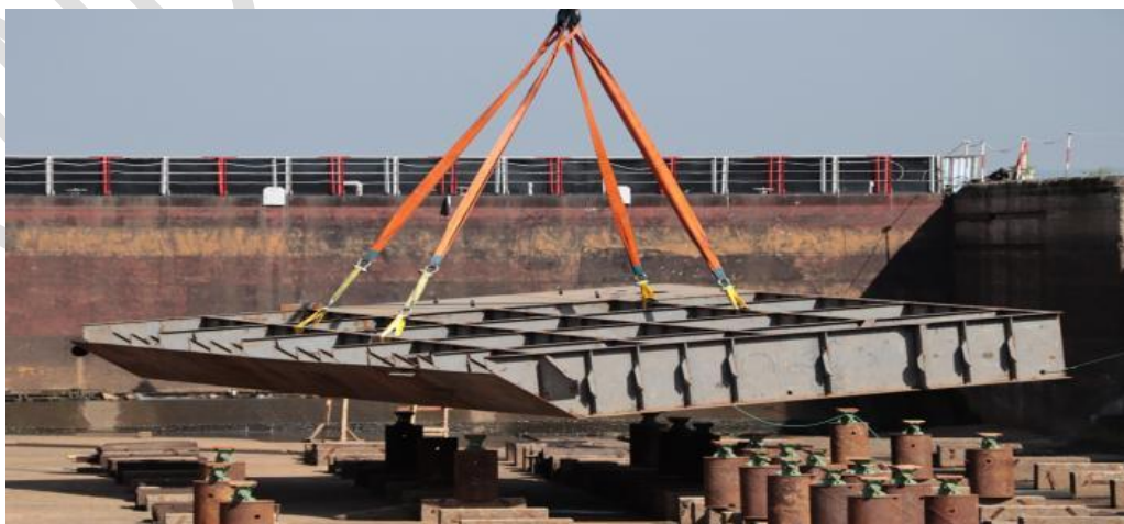
Fig-15 Installation of first section
