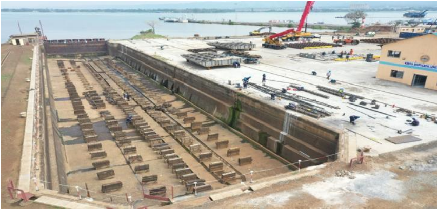
Fig-10 Fabrication of first hull section for MV Uhuru II wagon
