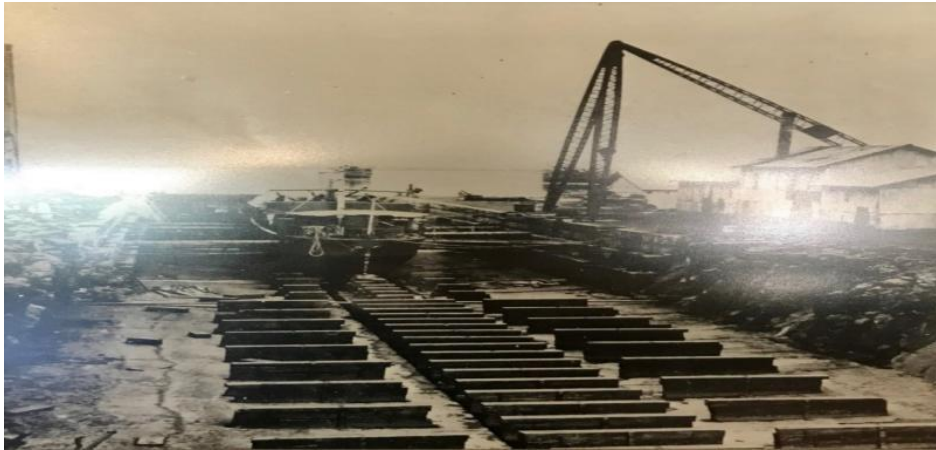
Fig -2 Dry dock during Construction period in 1905
