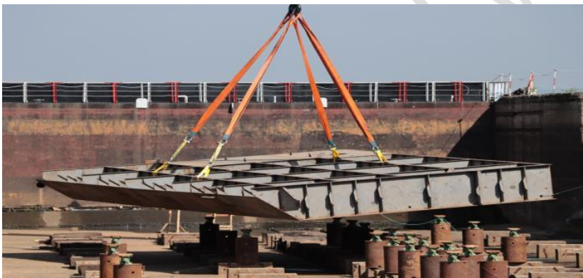
Fig-14 Installation of first section
