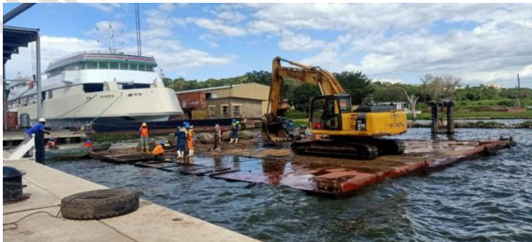
Fig-3 Dredging work at dry dock frontage
