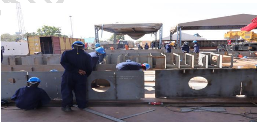
Fig-12 Fabrication of the sections
