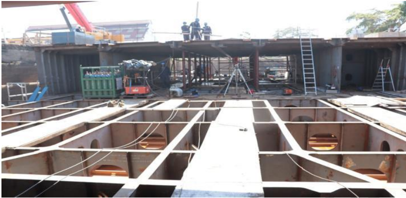
Fig-16 Installation of upper deck section
