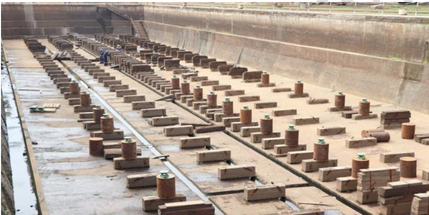
Fig – 11 Installation of Keel blocks and pipe stand
