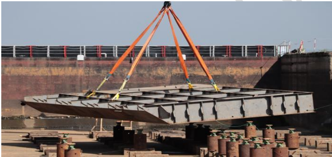
Fig-14 Installation of first section
