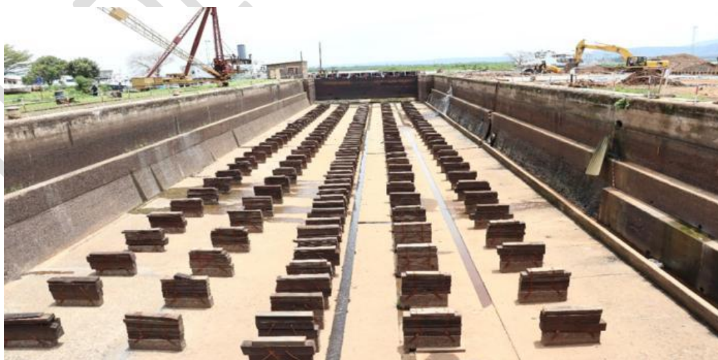
Fig-9 Preparation of dry Dock prior for MV Uhuru II Construction
