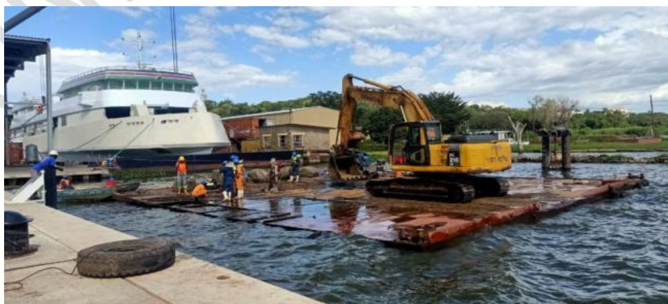
Fig-3 Dredging work at dry dock frontage
