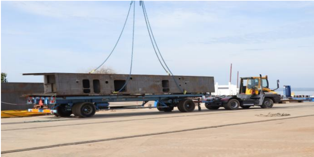
Fig -13 Transportation of sections from fabrication yards
