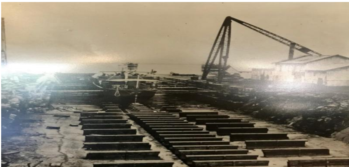
Fig -2 Dry dock during Construction period in 1905
