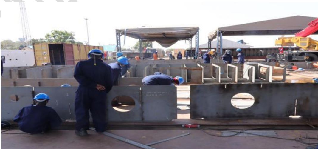
Fig-12 Fabrication of the sections
