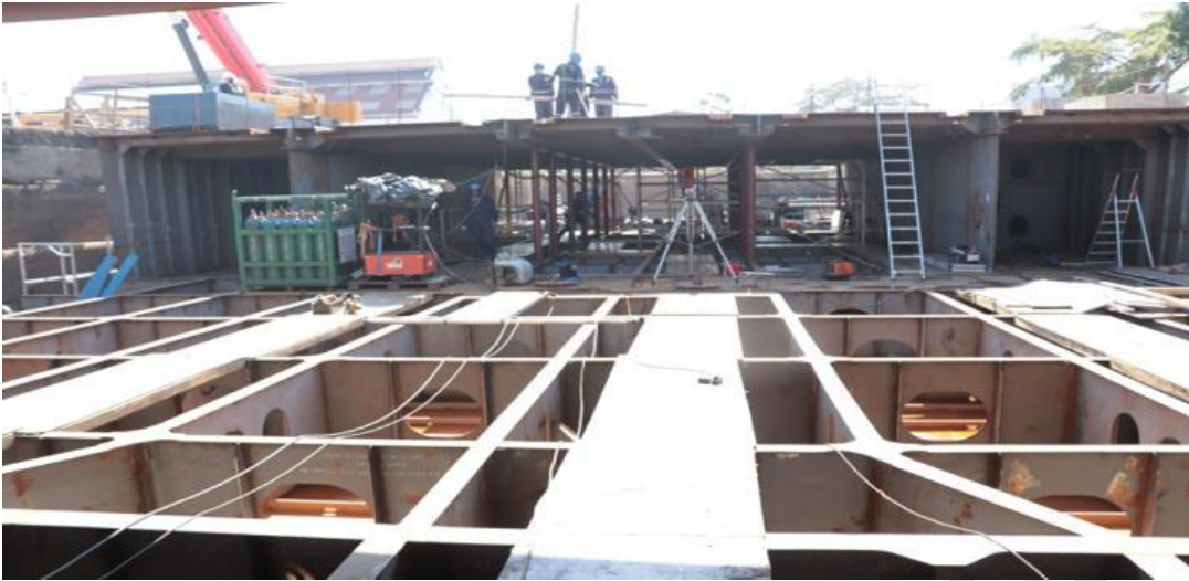
Fig-16 Installation of upper deck section
