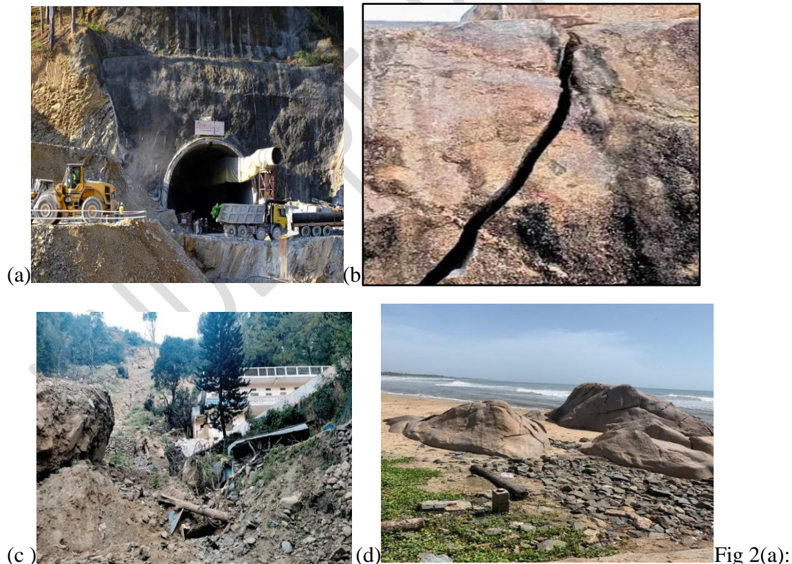
Fig 2(a): Tunnel subsidence UttarKasi Fig 2(b) Crack in Narasappa Konda hills, Kurnool (Fault induced) Fig 2(c): LS in Gaharwar Hills on 7 th Jan 2023, National herald; Chaturvedi, P. , Fig 2(d): Subsidence near shore temple Mahabalipuram (24.08.2023)
