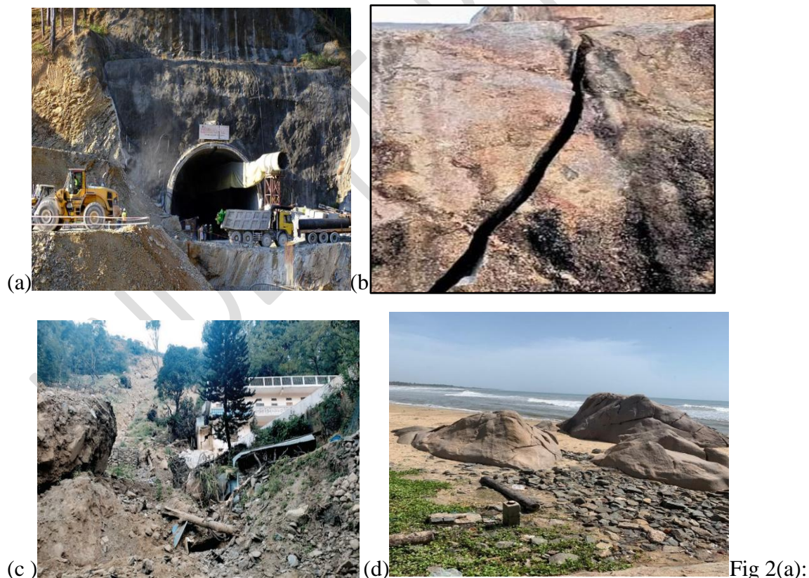
Fig 2(a): Tunnel subsidence Uttarakashi Fig 2(b) Crack in Narasappa Konda hills, Kurnool (Fault induced) Fig 2(c): LS in Gaharwar Hills on 7 th Jan 2023, National herald; Chaturvedi, P. , Fig 2(d): Subsidence near shore temple Mahabalipuram (24.08.2023)
