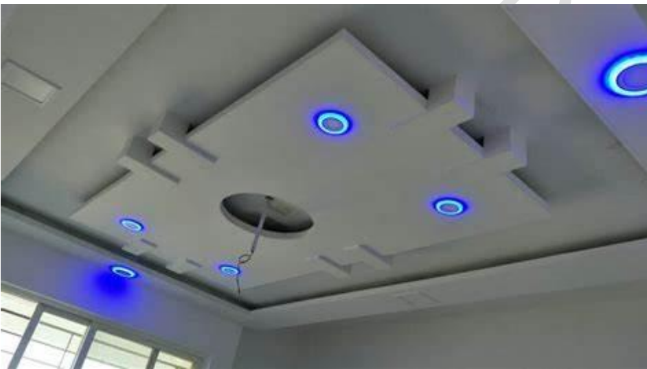
Fig. 2. POP ceiling finishing. Source: [7]
