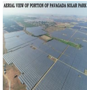
Figure 6. Solar Power Parks
