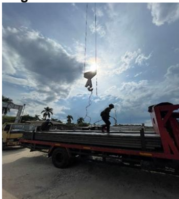
Figure 2. Material mobilization from stockyard to work site
