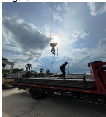
Figure 2. Material mobilization from stockyard to work site
