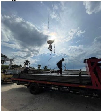
Figure 2. Material mobilization from stockyard to work site
