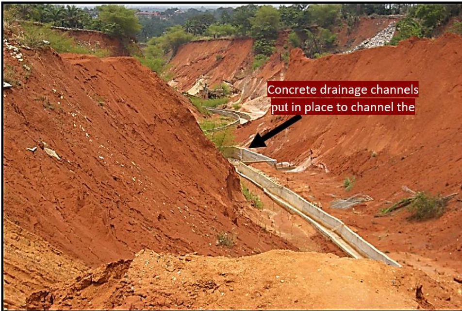
Fig 8: Control measure put in place to check gully erosion [1].
