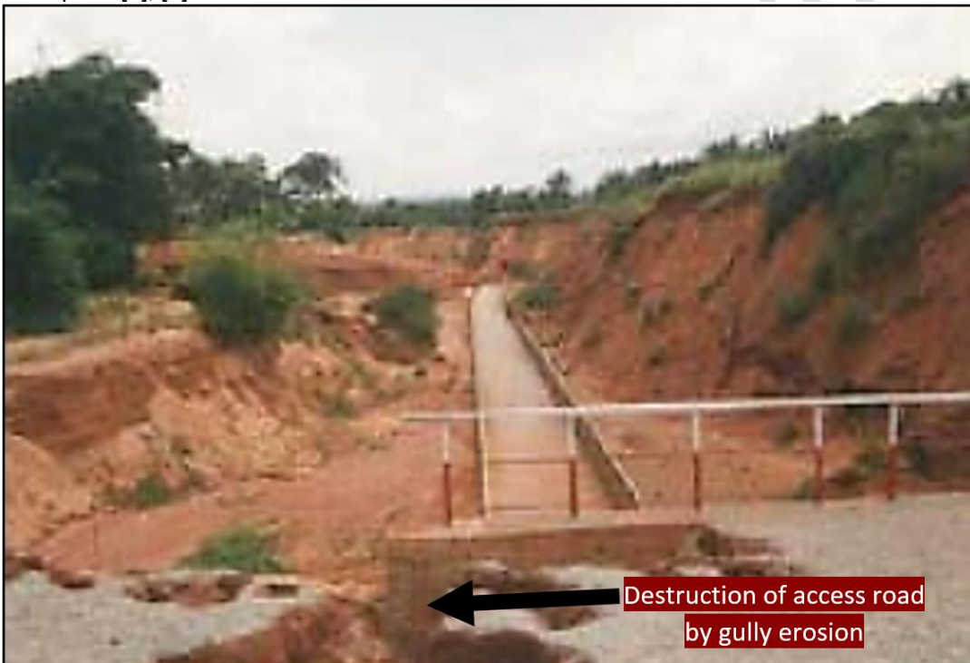
Fig 6: A Gully Site in Umuchiana, Aguata, showing the dissection of access road [12]
