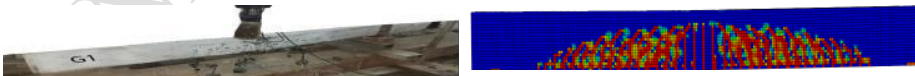
a) Cracking Patterns for Beam (G1) [EXP]. b) Cracking Patterns for Beam (G1) [FEM].
