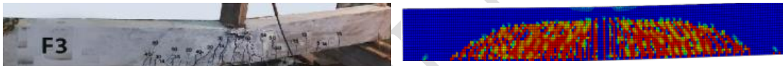
a) Cracking Patterns for Beam (F3) [EXP]. b) Cracking Patterns for Beam (F3) [FEM].
