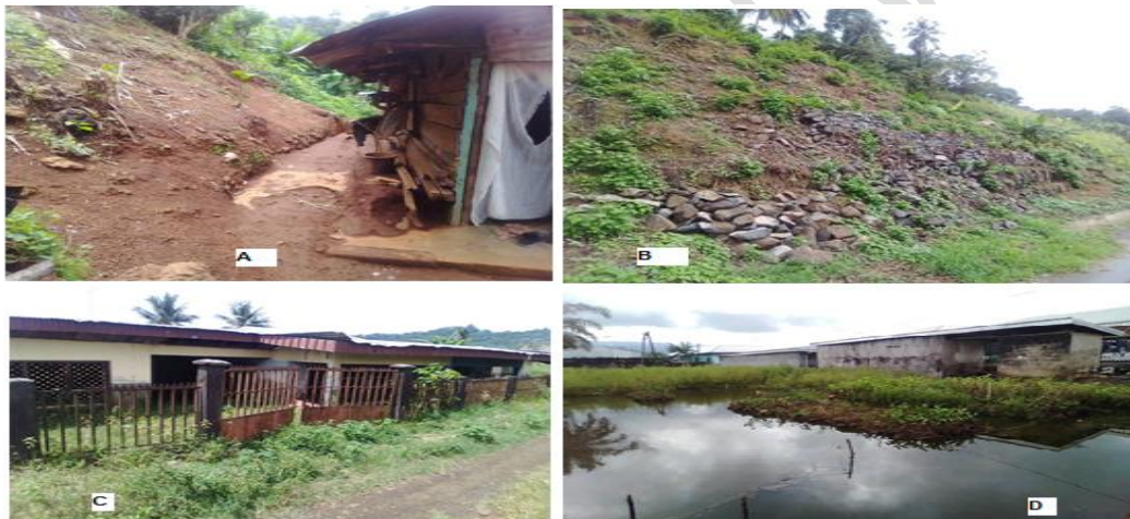
Plate 1. Some effects of hydrogeomorphic hazards Source: Fieldwork, 2022
