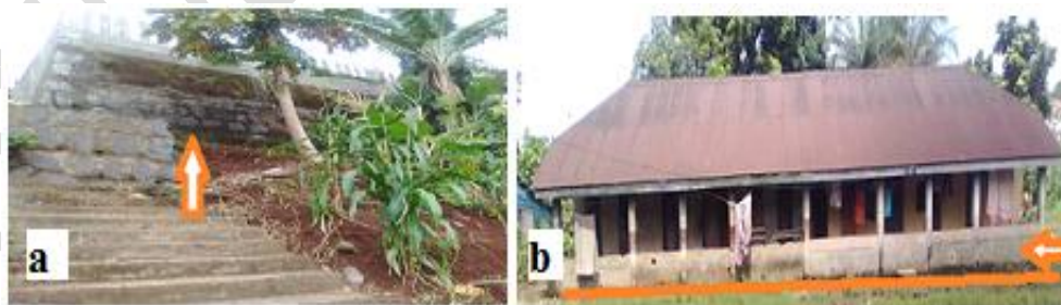
Plate 3. Other strategies against landslide and floods Source: Fieldwork, 2022
