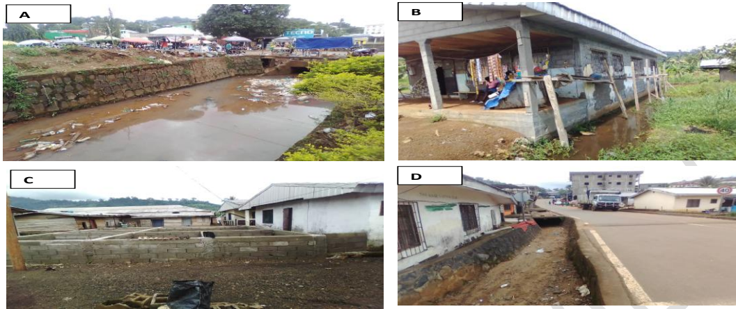
Plate 2. Some Flood control measures in Limbe Source: Fieldwork, 2022
