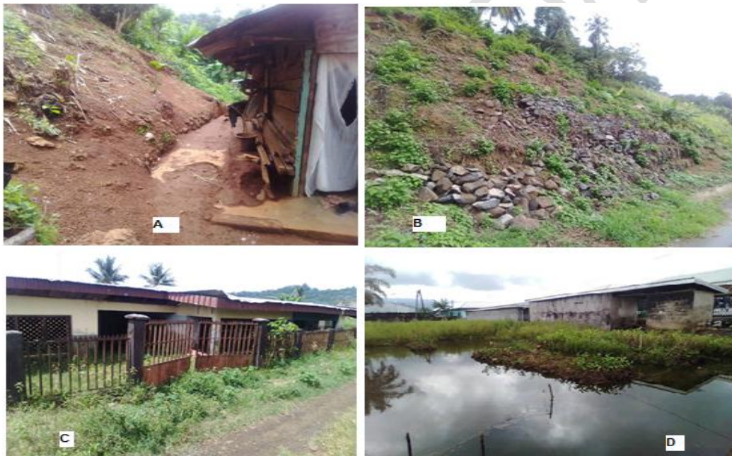
Plate 1. Some effects of hydrogeomorphic hazards Source: Fieldwork, 2022
