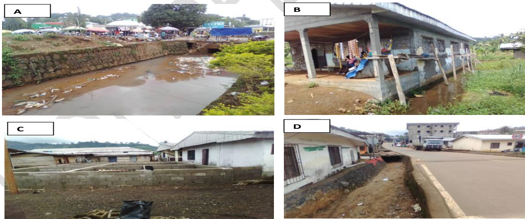
Plate 2. Some Flood control measures in Limbe.
