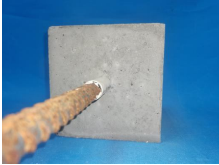
Fig. 2 .Pull Out Damage
