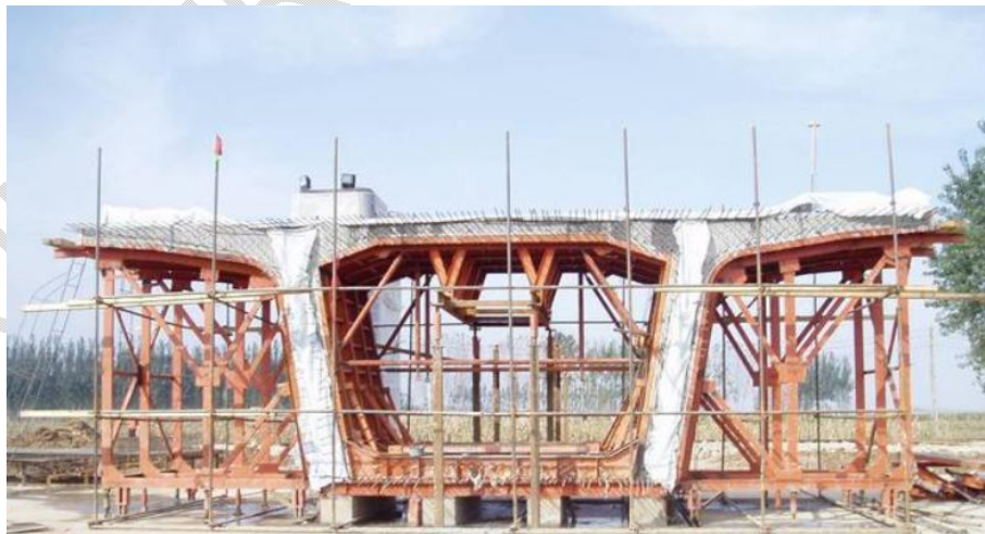
Fig.7 Construction drawing of formwork removal
