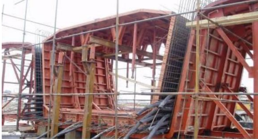
Fig.6 Formwork installation construction drawing
