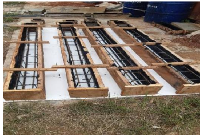
Figure 4: Wooden formwork for Beams
