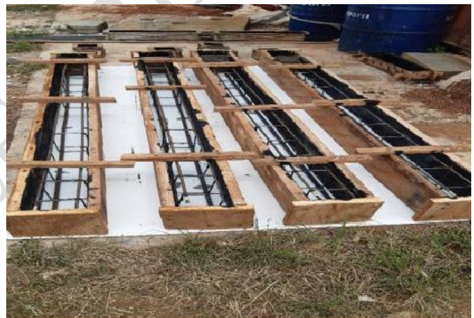
Figure 4: Wooden formwork for
