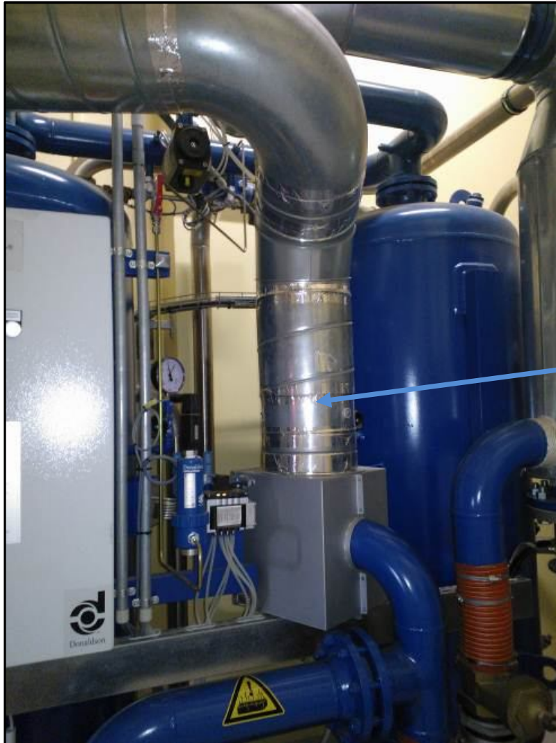
Figure 5: Heat recovery between compressor and dryer
