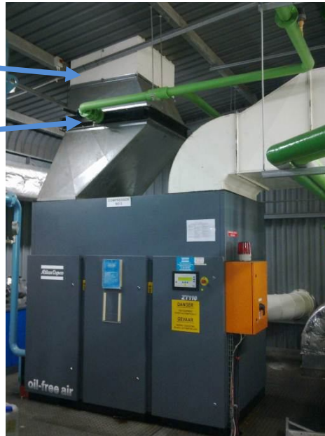
Figure 9: Example of heat recovery on a compressed air to produce hot water thanks to an exchanger
