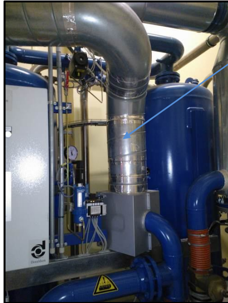
Figure 5: Heat recovery between compressor and dryer
