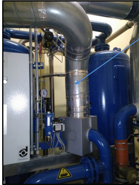
Figure 5: Heat recovery between compressor and dryer
