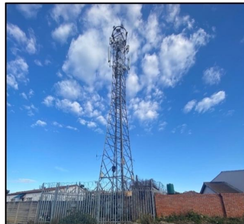
Fig. 13. Telecommunication towers built near houses
