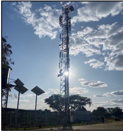
Fig. 14. Telecommunication towers built near municipal facilities
