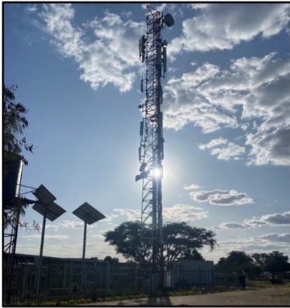
Fig. 14. Telecommunication towers built near municipal facilities
