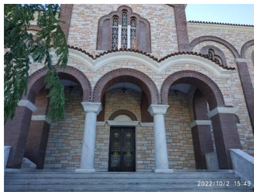
Figure 19. A Non-linear structure (Church) in a natural environment with few trees and without PnP linear geometries → No Birds’ nests found.
