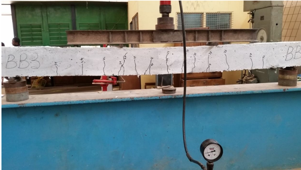
Figure 5: Crack propagation and characteristics of the 0.25% fibre concrete
