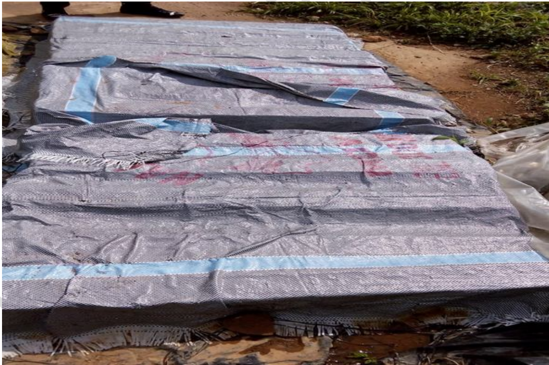
Plate 1: Curing of Experimental Beams.
