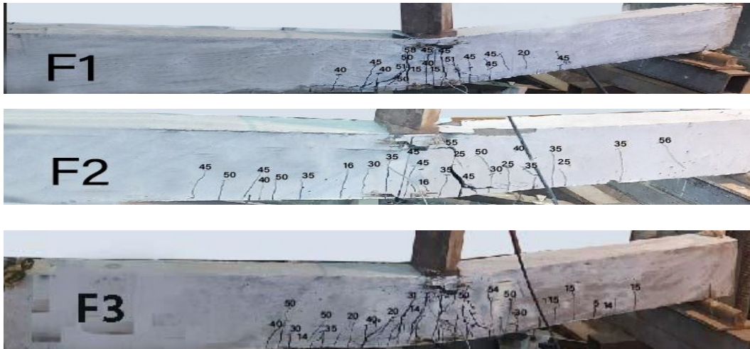
Fig (26): Cracking Patterns for Group (F).
