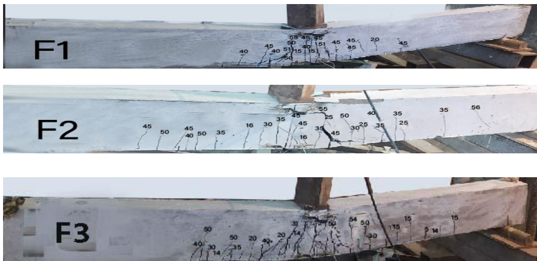
Fig (26): Cracking Patterns for Group (F).
