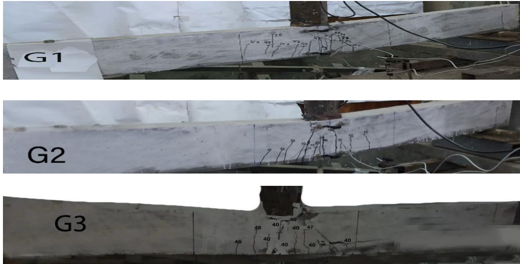
Fig (25): Cracking Patterns for Group (G).
